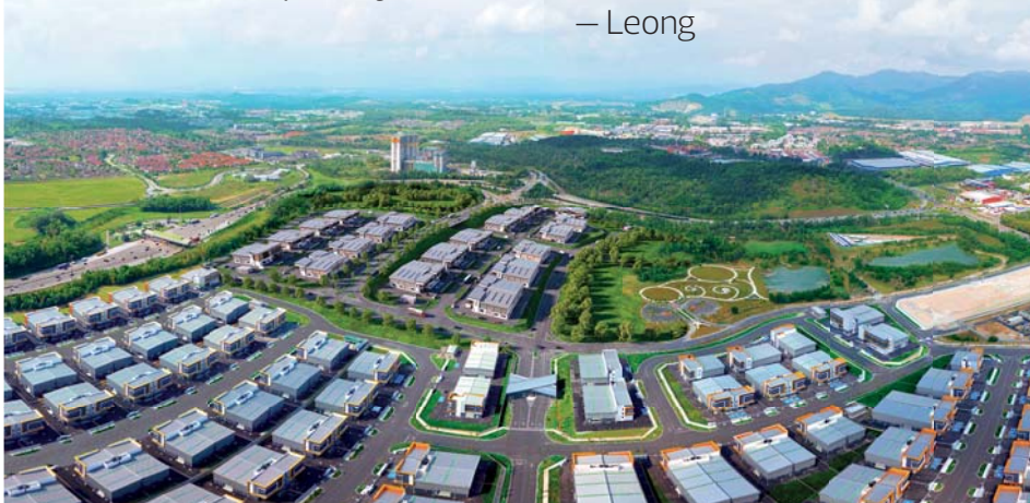
XME Business Park offers ready-built factories and has easy access to the NSE and KLIA via the upcoming NLE
