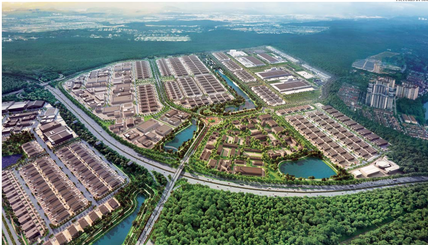
Elmina Business Park 2 is the next-generation extension of high-quality, ESG-oriented industrial parks with strategic connections to three major expressways – the GCE, NSE and LATAR
