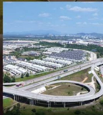
Infrastructure Gerbang Nusajaya Interchange
